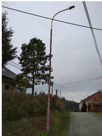
Obr. 7 Stožár mimo osu
